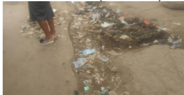
Plate 4: Existing block drainage
