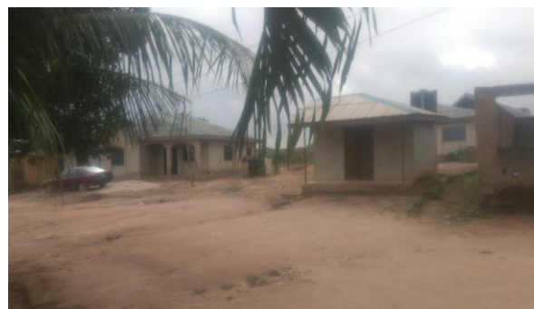
Plate 8: Street without drainage and untarred
