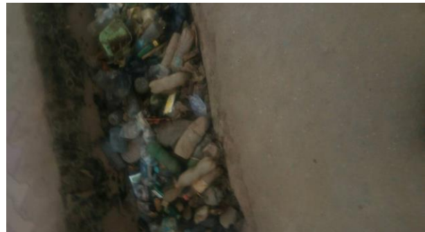
Plate 5: Existing block drainage
